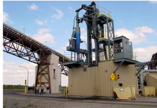
Automated Truck Auger
